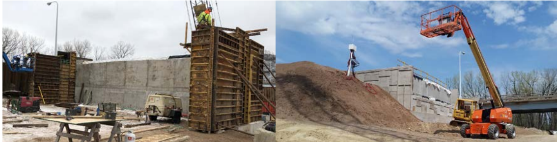
Figure 3. Construction of the north abutment is shown (at left) prior to embankment backfilling. At right, new fill can be seen to the left of the abutment. The bridge beams are not yet placed.
